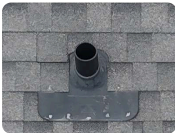
Plumbing vent and flashing
